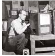
Worker checking television wiring
