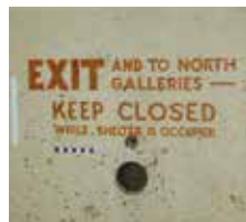
Exit sign underground shelter ARS1 Blast door
