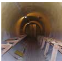
One of the tunnels in the factory's underground shelter
